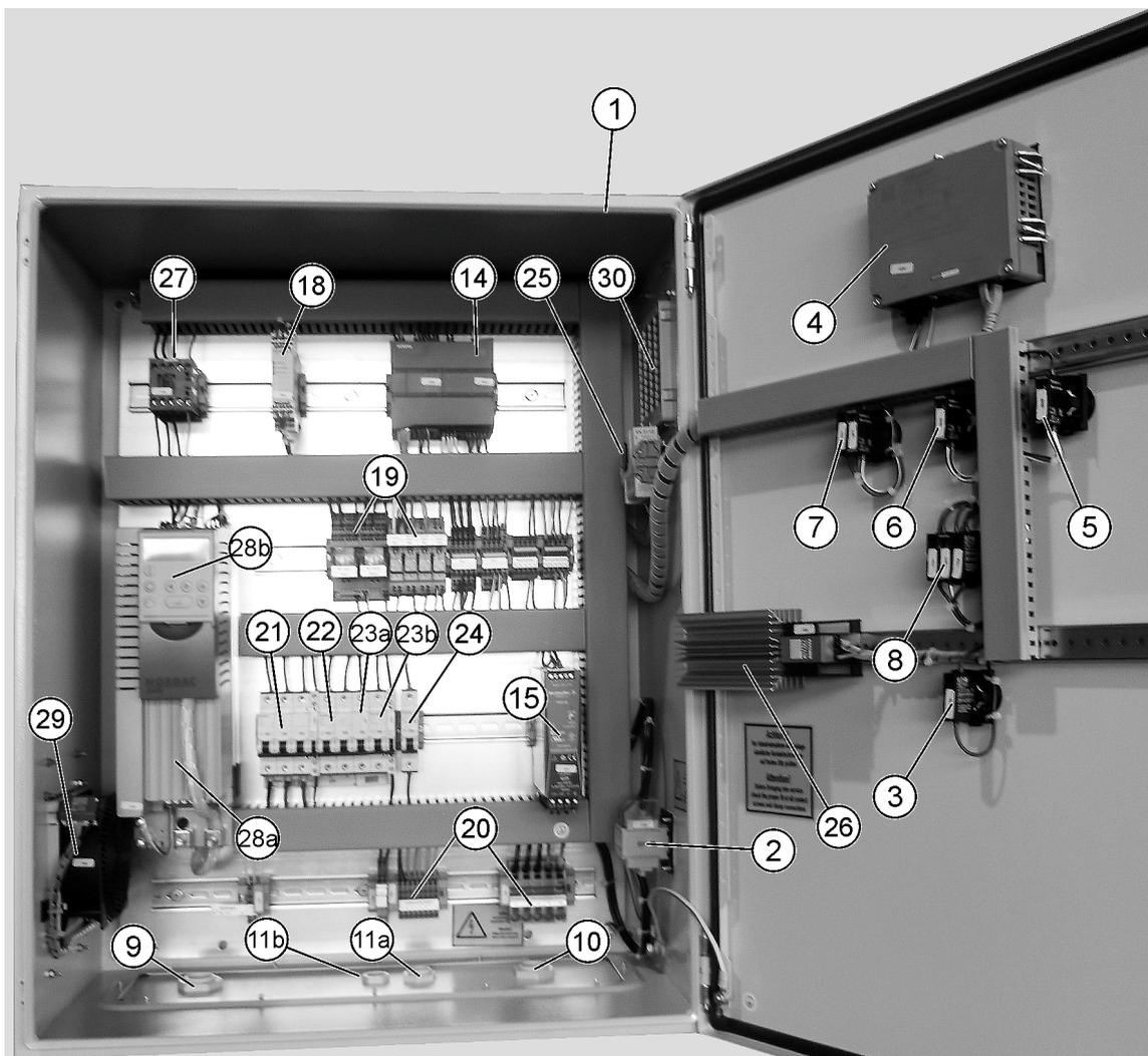
Inside of the control cabinet, version with frequency converter
