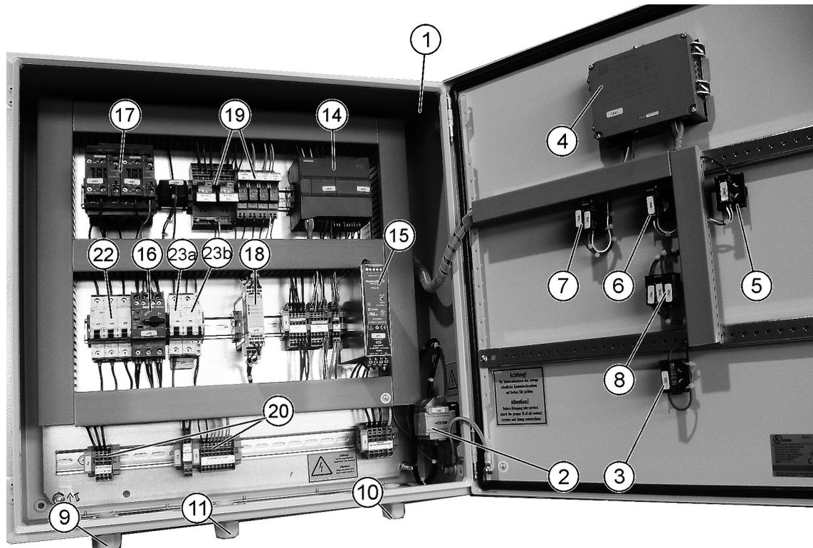
Inside of the control cabinet, version with reversing contactor combination and motor protection switch
